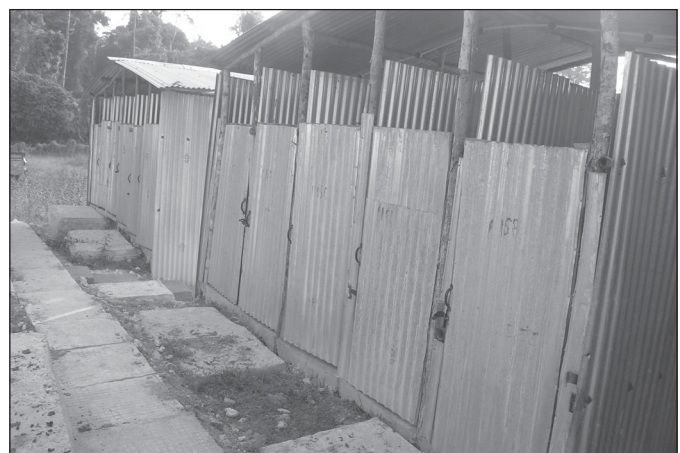
Poorly constructed toilets with low doors and incomplete walls, PHC shelter
