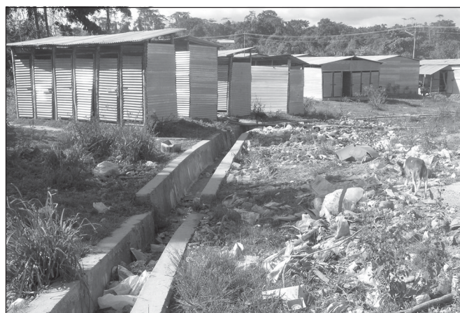
Uncovered drains and absence of solid waste management facilities at PHC shelter
