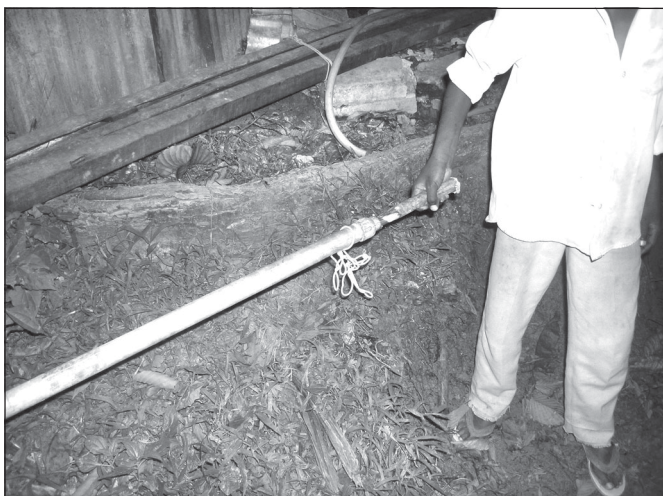
Inadequate outlet for piped water in Panchu Tikree
