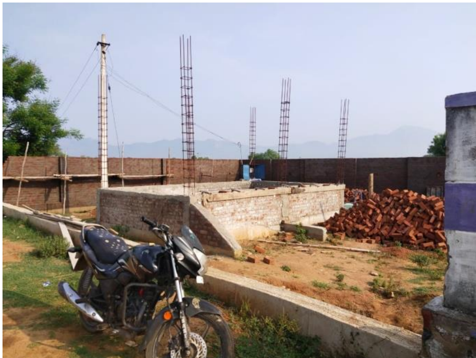
Construction of cremation ground in the settlement of Soolapuram, Madurai
