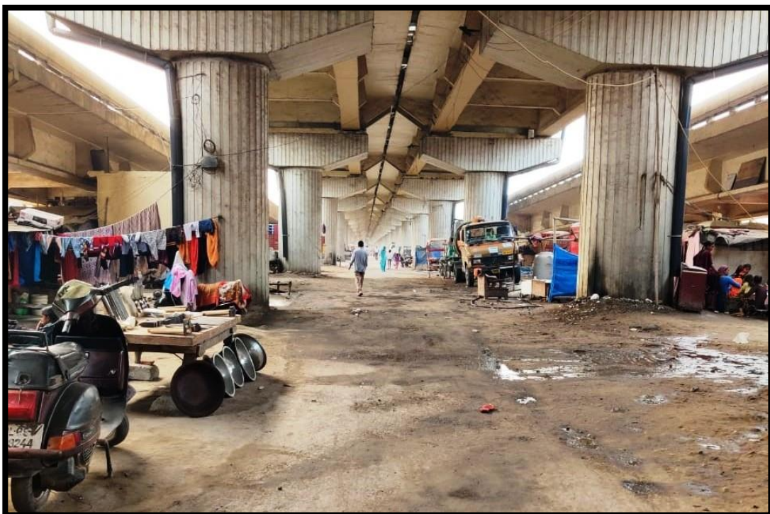
The settlement under the flyover in Mansarovar Park, Shahdara
