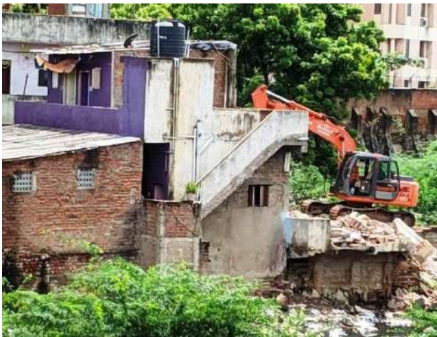
Demolition in Kakkan Nagar, Chennai
