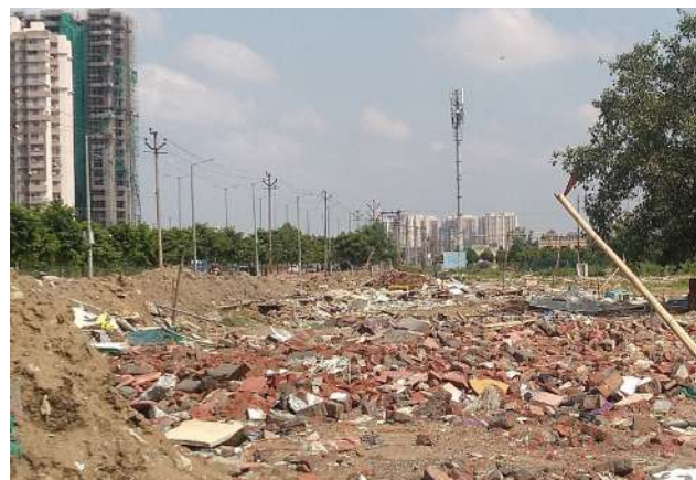
Demolished houses in Sector 116, Noida
