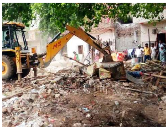
Demolition in Mansarovar Park, Delhi
