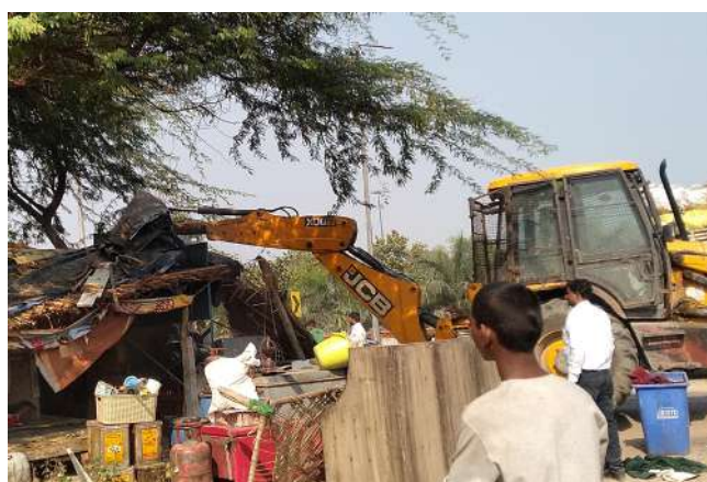
Demolition underway in New Ashok Nagar, Delhi
