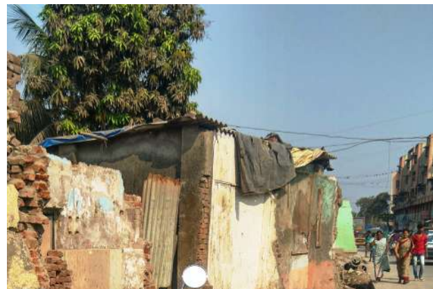
Demolished houses and shops near Panvel Flyover, Navi Mumbai
