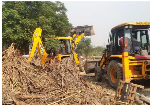
Demolition drive underway along the banks of the Yamuna River
