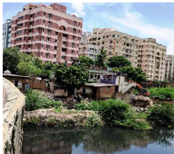
Houses being demolished along the banks of the Cooum River in Chennai
