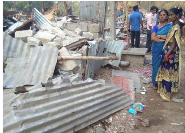
Houses demolished in Yari Road, Versova, Mumbai
