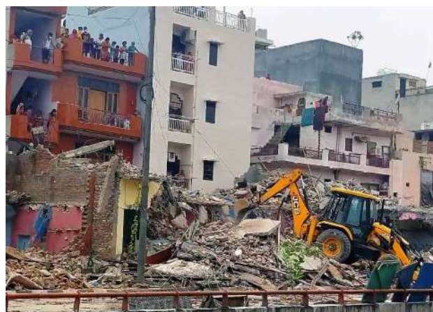
Demolition drive at East Laxmi Market, Delhi
