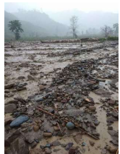
Asian Development Bank-sponsored road project in Phalong
